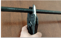
Step 1: Cut Unipro Metco Pipe at 90° angle
